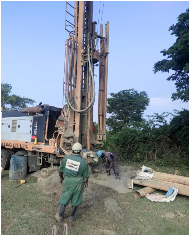
Borehole drilling at Kanyamfwa Secondary School
